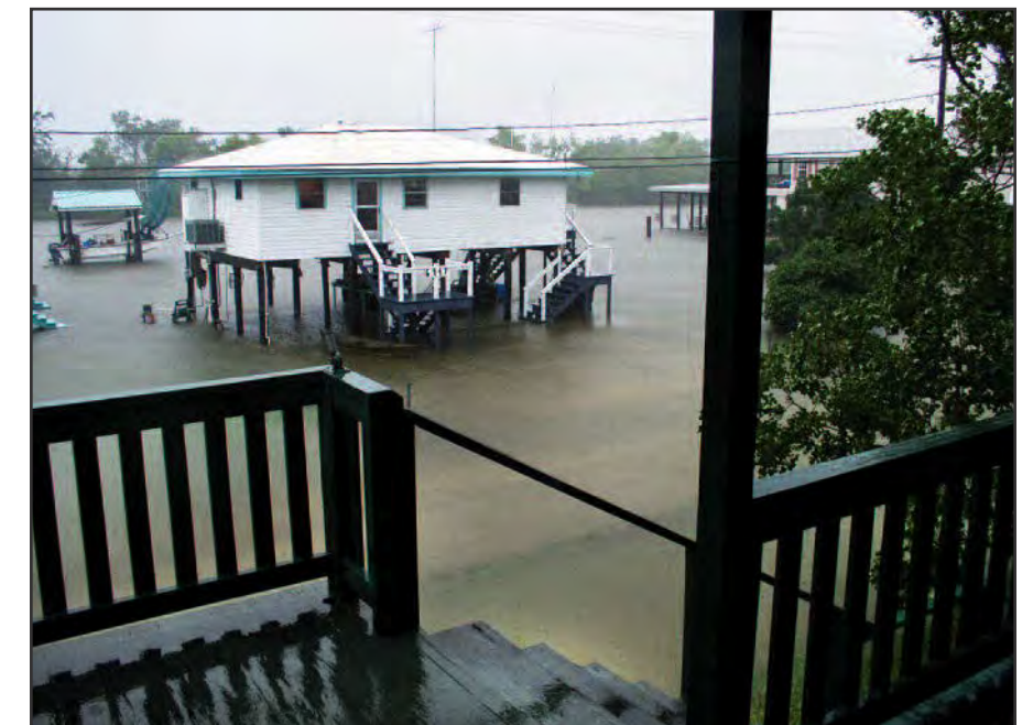
Houses in Louisiana's southernmost communities are built on stilts for a reason, as evidenced in Cocodrie during Tropical Storm Bill in 2007. Photo: © sleepyorange via Flickr
